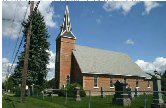
Plate 4: St. David's Anglican Church, County Road 13.
