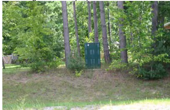
Plate 10: Buried utilities located within the residential areas.
