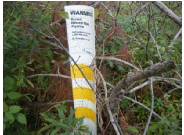
PLATE 38 NATURAL GAS LINE MARKER
