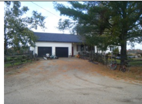
PLATE 34 HOUSE AND GRAVEL LANE
