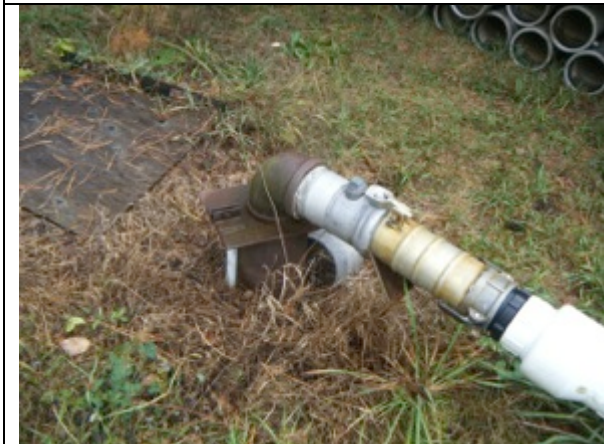
PLATE 41 IRRIGATION HOOK UP
