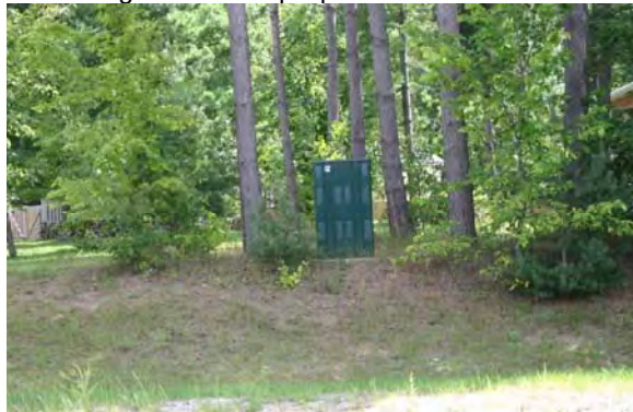
Plate 10: Buried utilities located within the residential areas.
