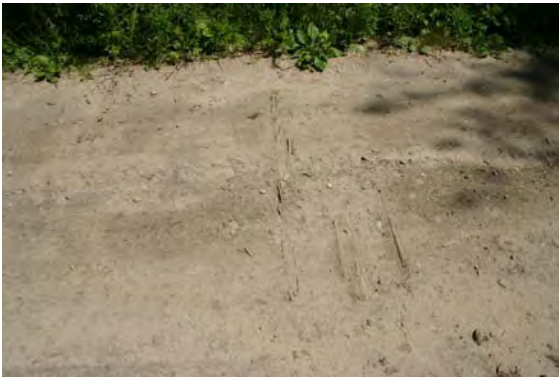
Plate 41: Corduroy Road within Concession Road 6.
