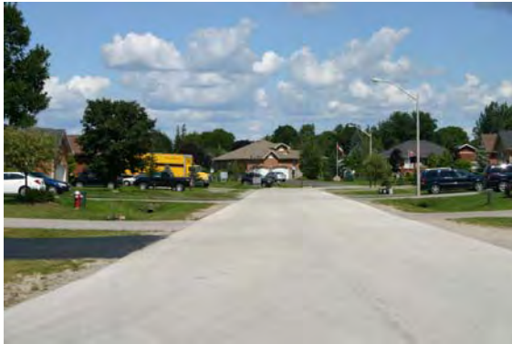
Plate 43: Typical roadway and right of way within the residential areas.
