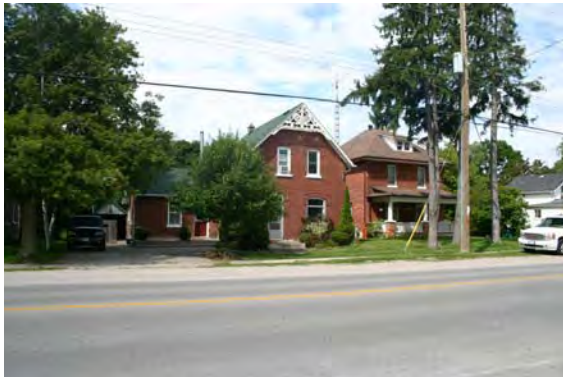
Plate 3: The late-nineteenth and early twentieth century structures within the settlement area of Everett.
