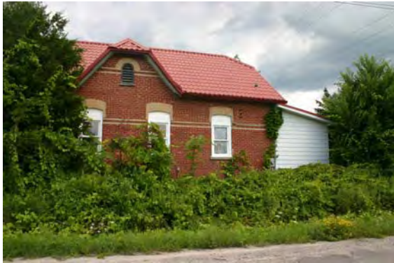
Plate 19: The residence at the intersection of Concession Road 4 and County Road 5.
