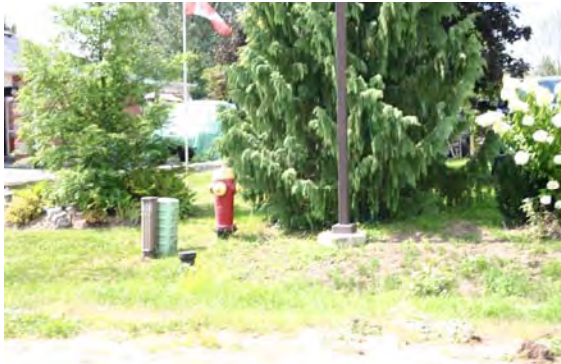
Plate 45: Typical utilities encountered in the right of way along the residential roads.
